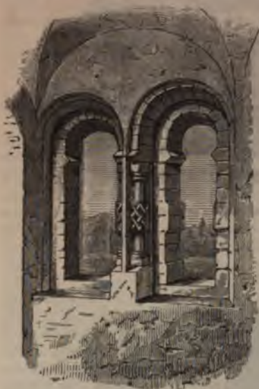
NORTH WINDOW, GREAT TOWER, RISING CASTLE.
